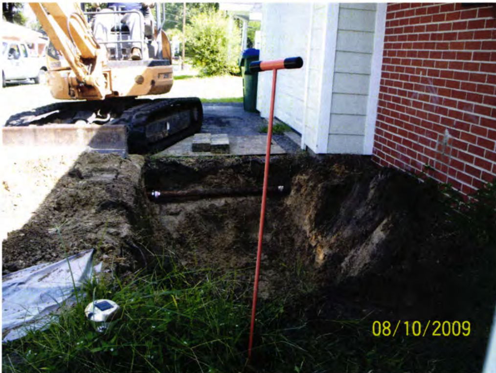
Picture 2: UST 1456Cardinal removal in progress.
